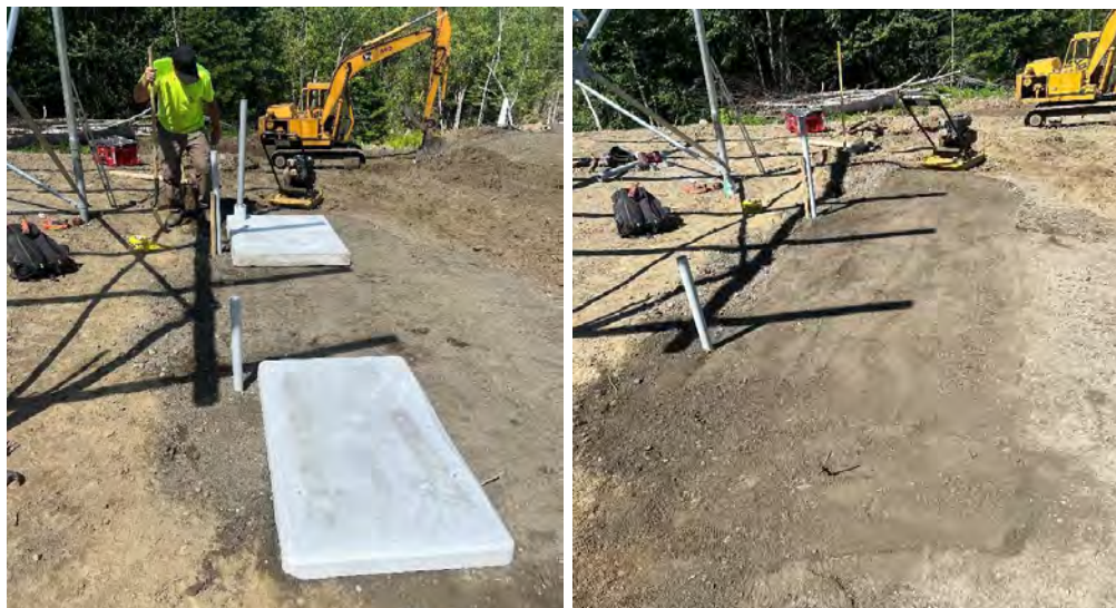
Figure 2 - Locating and placement of RaVolt enclosure pad
