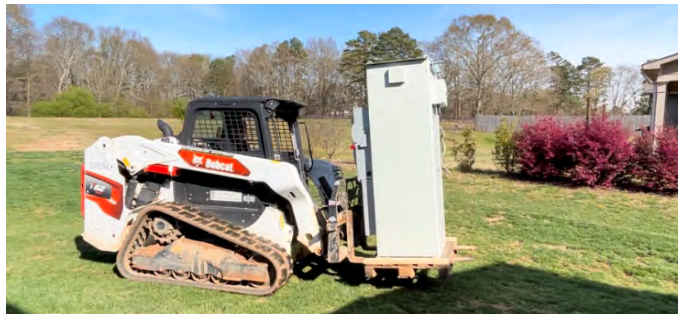
Figure 1 - Cabinet installation using excavator
