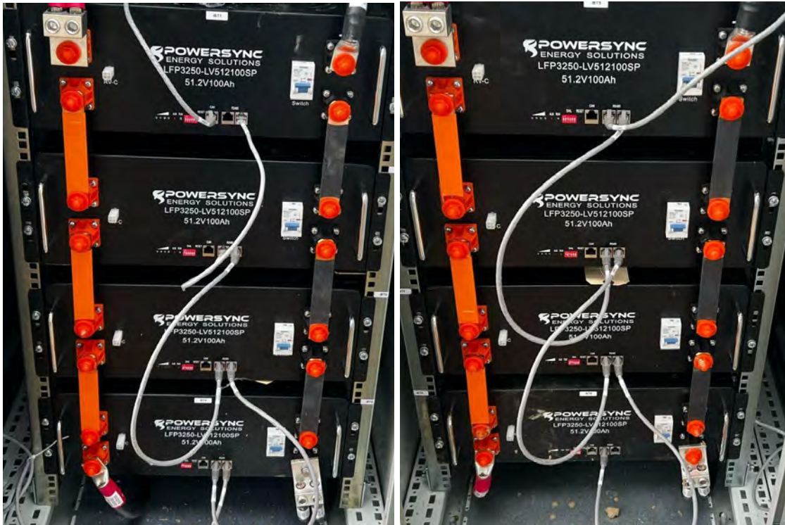
Figure 7 - Left side is the Master Cabinet, Right side is the slave cabinet.
