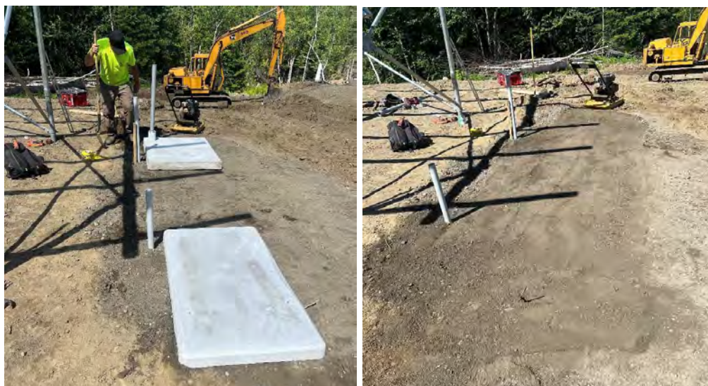
Figure 2 - Locating and placement of RaVolt enclosure pad
