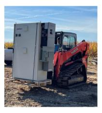
4. If using a mini excavator for unloading the equipment, utilize properly weight rated slings and properly weight rated shackles. The unit will arrive with 4 lifting points present on the top of the enclosure. Operator must use extreme caution to not bend or break these lifting points, which may interfere with the enclosure's NEMA 3R rating. If using a forklift
